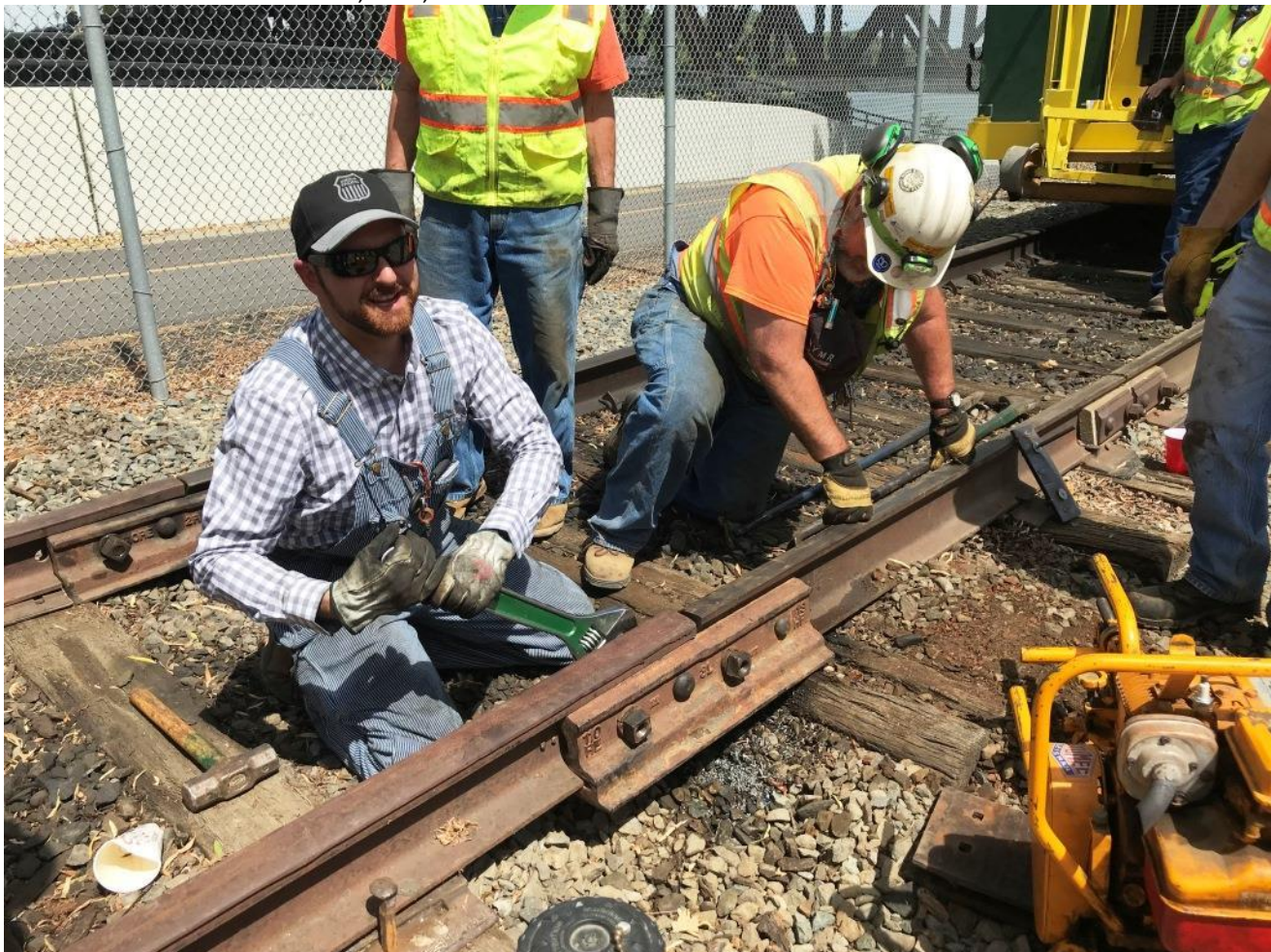
With the holes successfully drilled, Chris and Mike F. get the joint-bar bolted on
