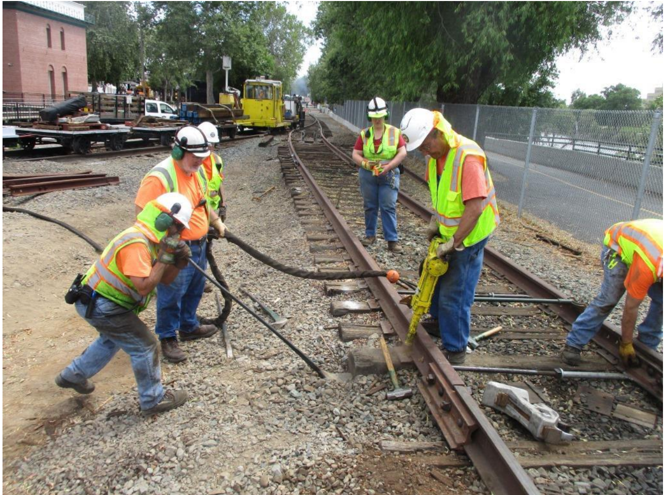
Frank handles the hydraulic hose for John, who takes on the hydraulic spike-driver as Joe nips up the tie
