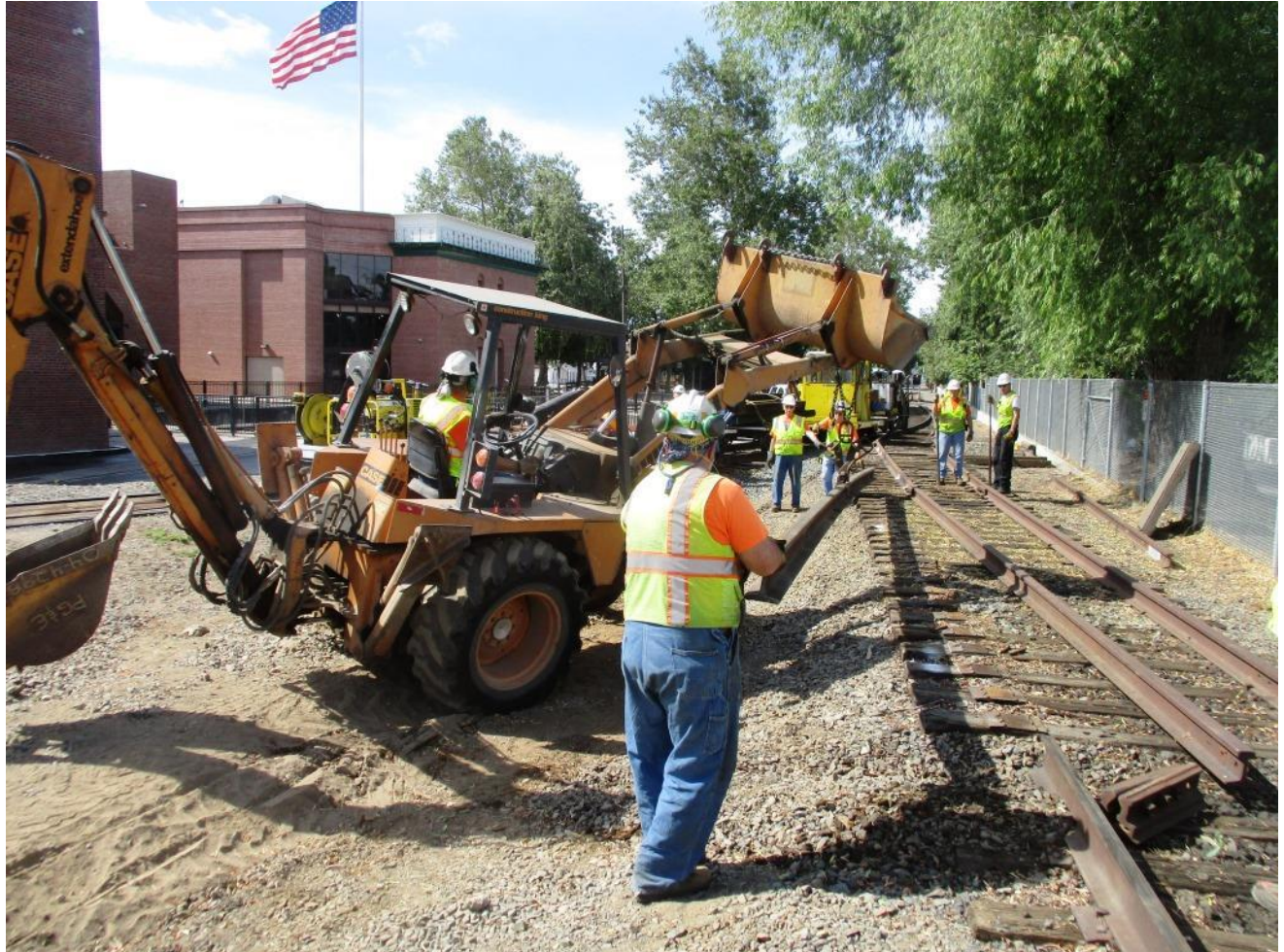
Mike F. guides another stick of 113-pound rail as it is hauled away
