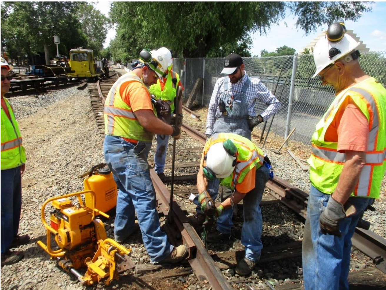
Mike F. and Joe get the bolts tightened down
