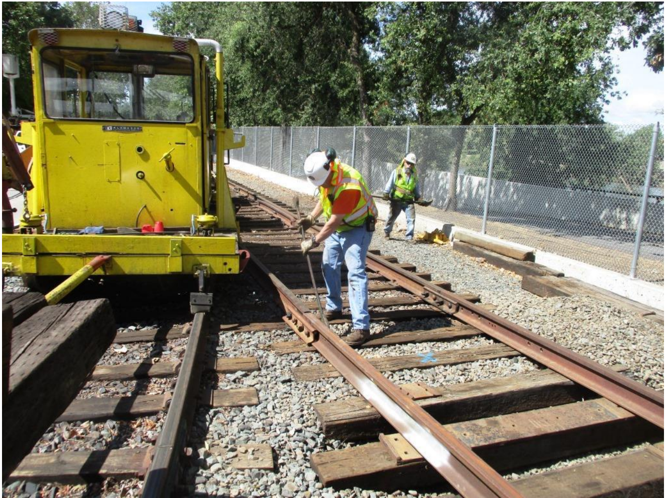
Bill tightens bolts at the south joint
