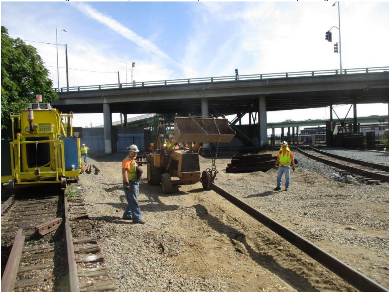
Ed on the back-hoe pulls a stick of 113-pound rail out of the way
