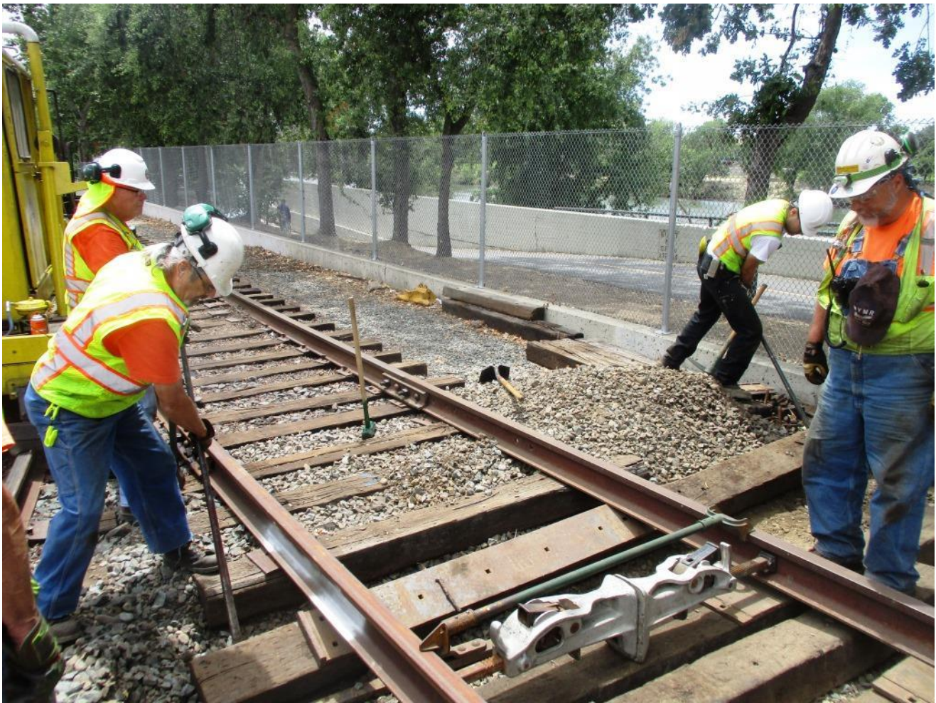
Ed and Kyle shimmy the head-block to the side to make room for digging out the west side
