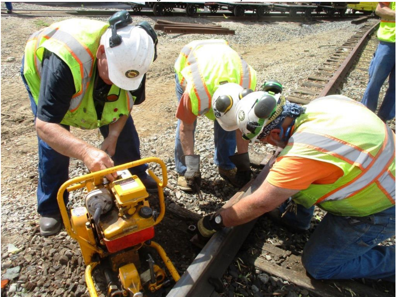
Harry, Clem, and Mike F. get the joint-bar in place to use as a template for drilling new bolt holes in the north rail
