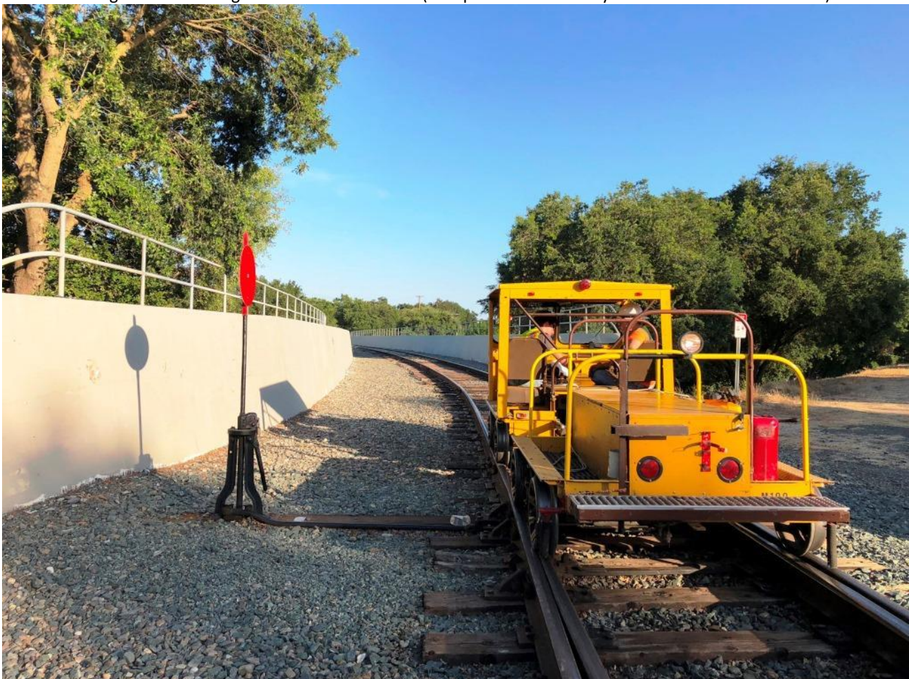
Jack and Mike H. in the MT-14 pass the newly restored switch target at Switch 20
