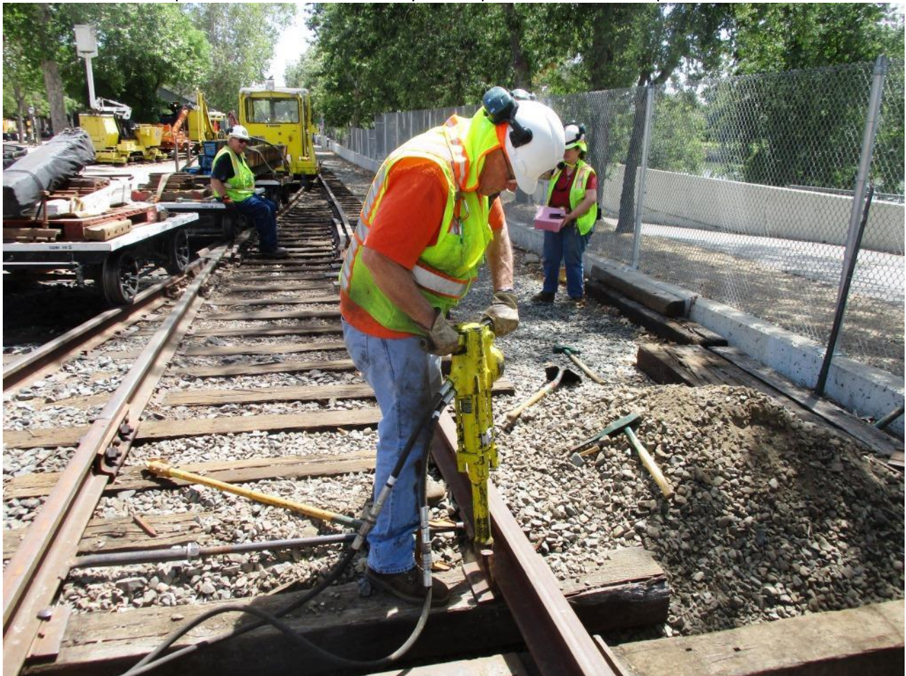
Bill drives spikes with the hydraulic spike-driver
