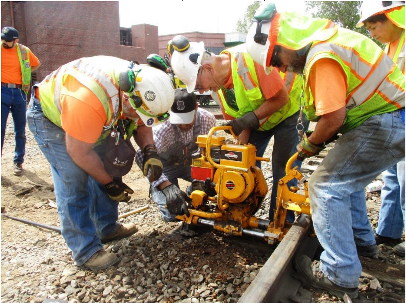
Mike F., Chris, Clem, and Joe line-up and level the heavy and unwieldy rail-drill
