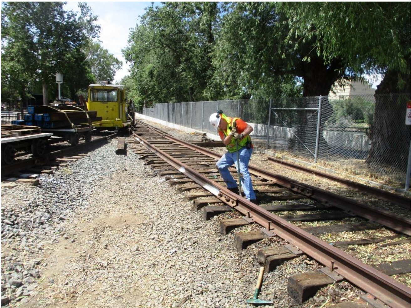
Bill tightens the bolts at the next joint south
