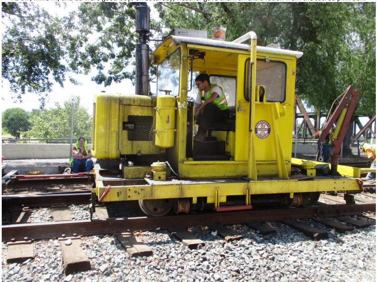
Kyle moves the Kalamazoo and work-train so as to deploy the hydraulic spike-driver
