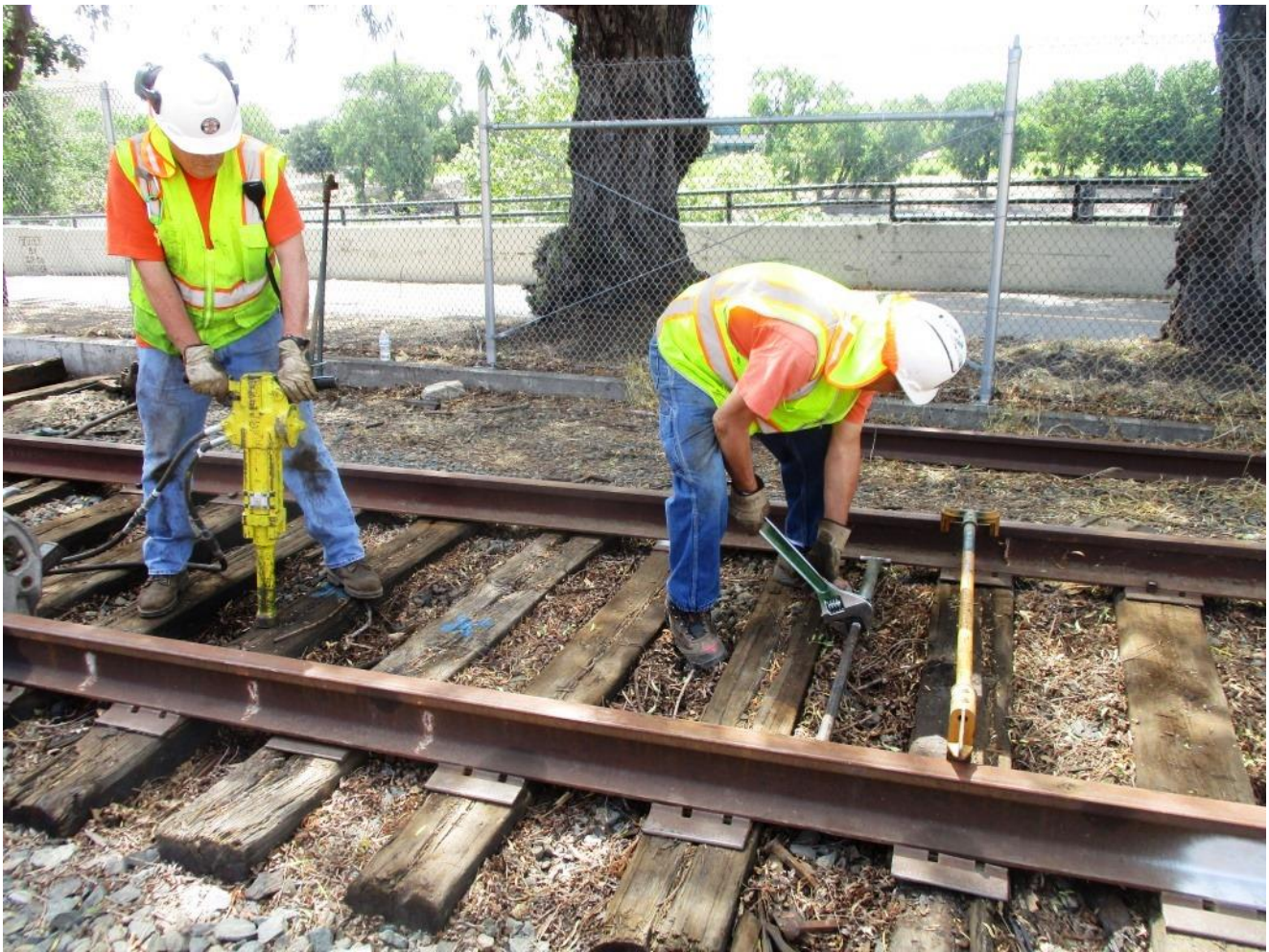
John spreads the rails apart until they are in the proper gauge
