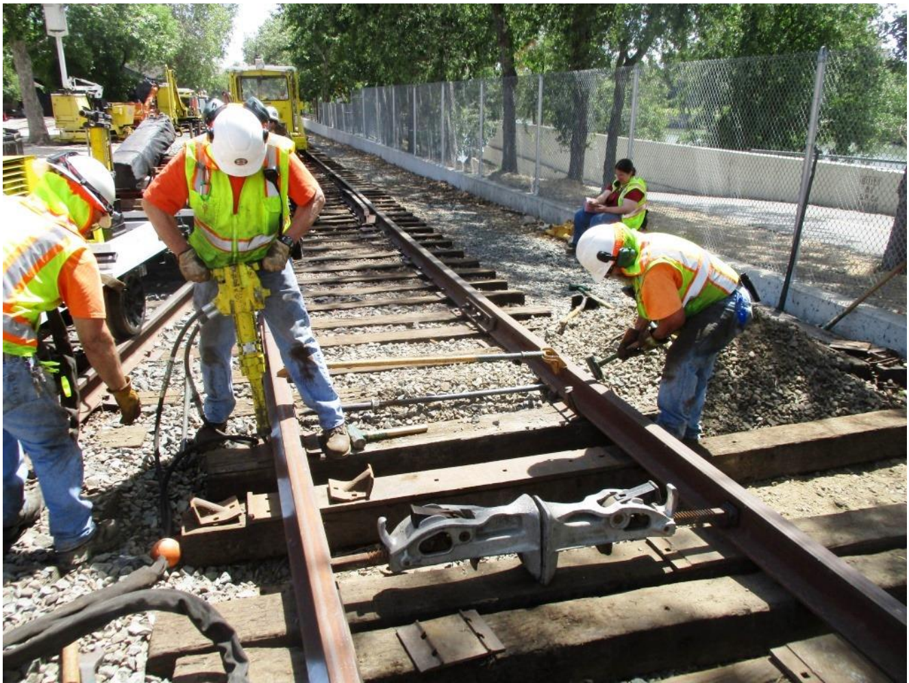
Bill drives spikes on the east rail with the hydraulic spike-driver as Joe sets spikes on the west rail
