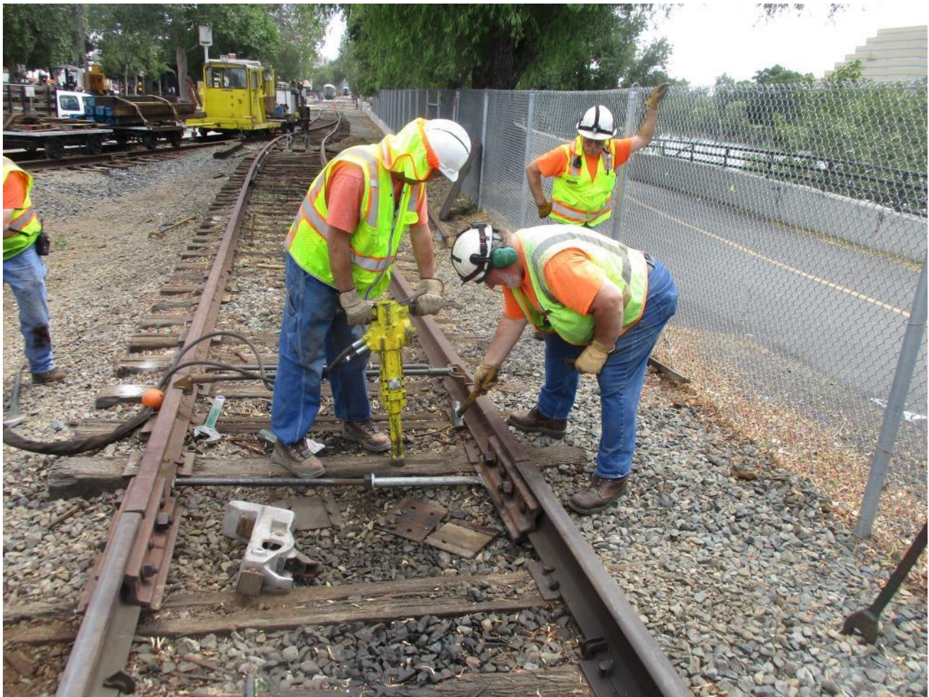
Frank knocks the tie-plate into position for John to drive the last spike of the day
