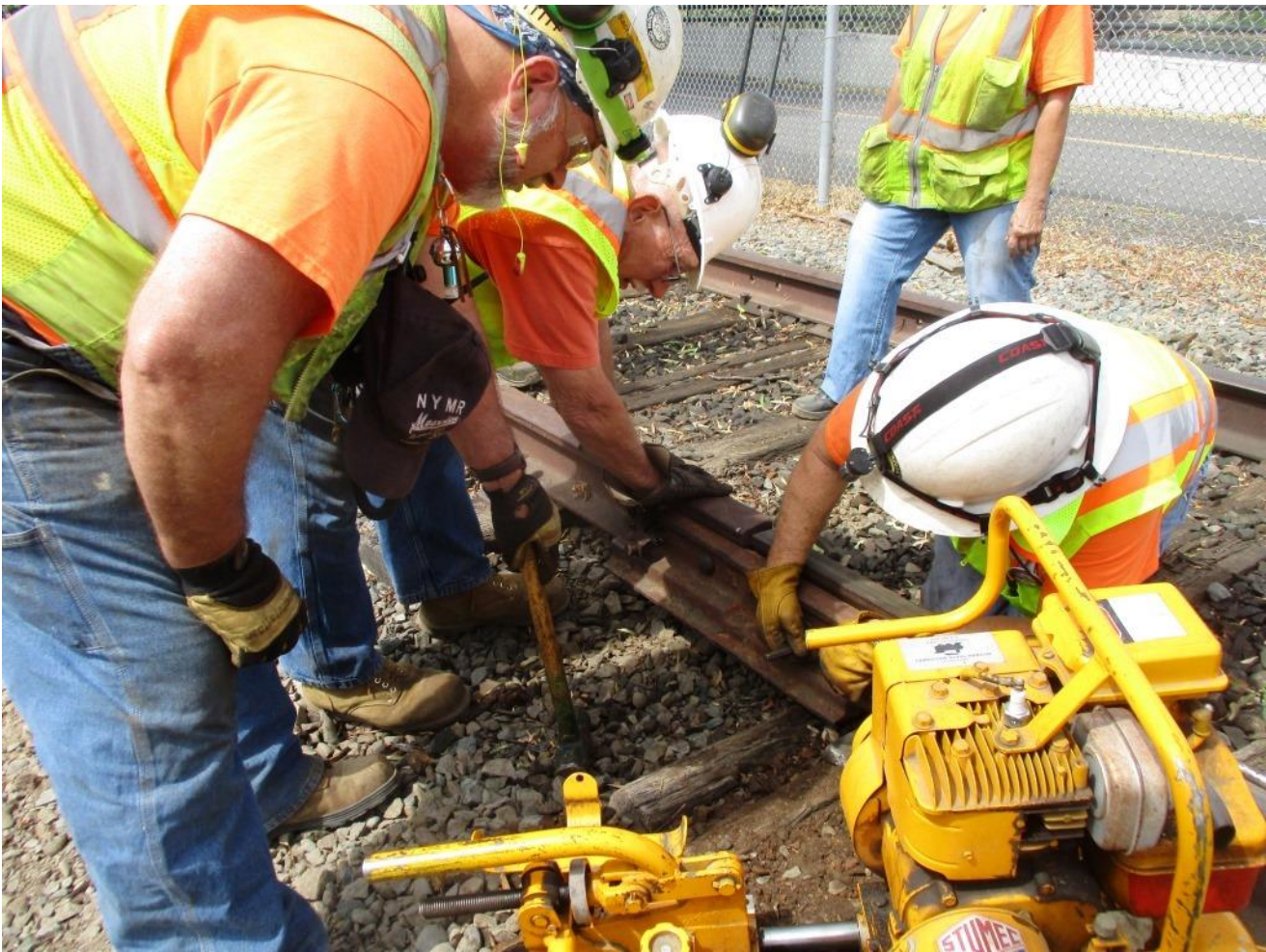
Mike H. uses a punch to mark the drill spot
