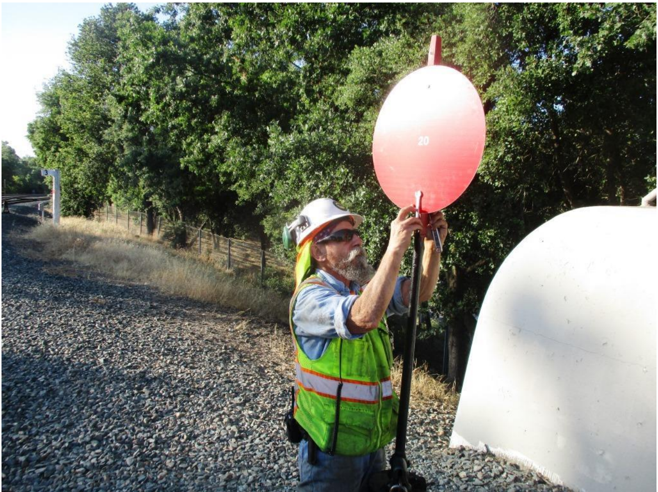
Joe gets the new target at Switch 20 installed (to replace that stolen by miscreants and malcontents)
