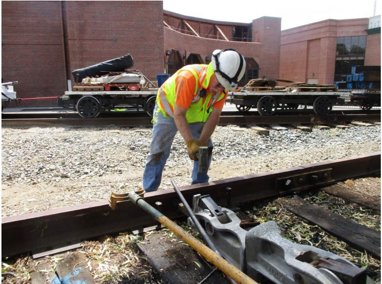
With this segment of the track in gauge, Mike H. sets spikes
