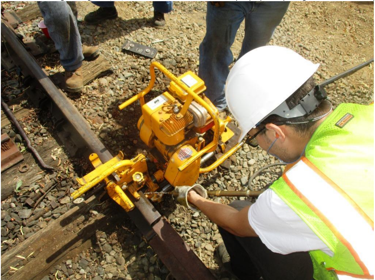
Kyle sprays water on the spinning drill-bit as it cuts a new bolt-hole in the web of the rail
